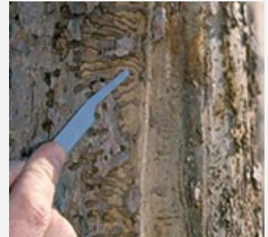
Vertical galleries with perpendicular branches (1).
