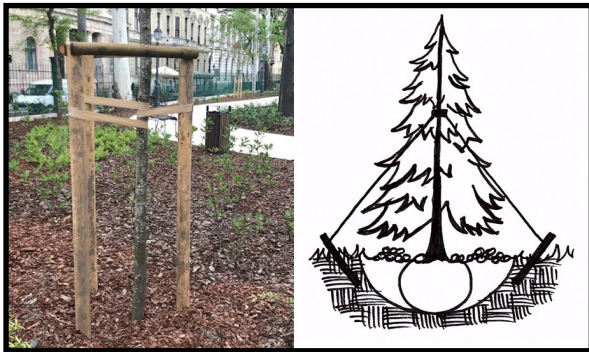
Figure 14. Three stakes, all larger than the tree trunk with pretty aggressive attachments ( left photo ) are designed to discourage vandalism to the trees ( a Jim Blake photo ). Larger trees, especially evergreens ( right ), commonly require a three anchor stake system for stability.
