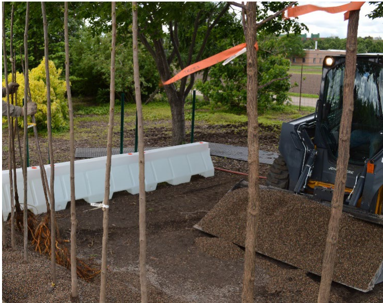
Plastic temporary traffic barriers used in a three-sided gravel bed.
