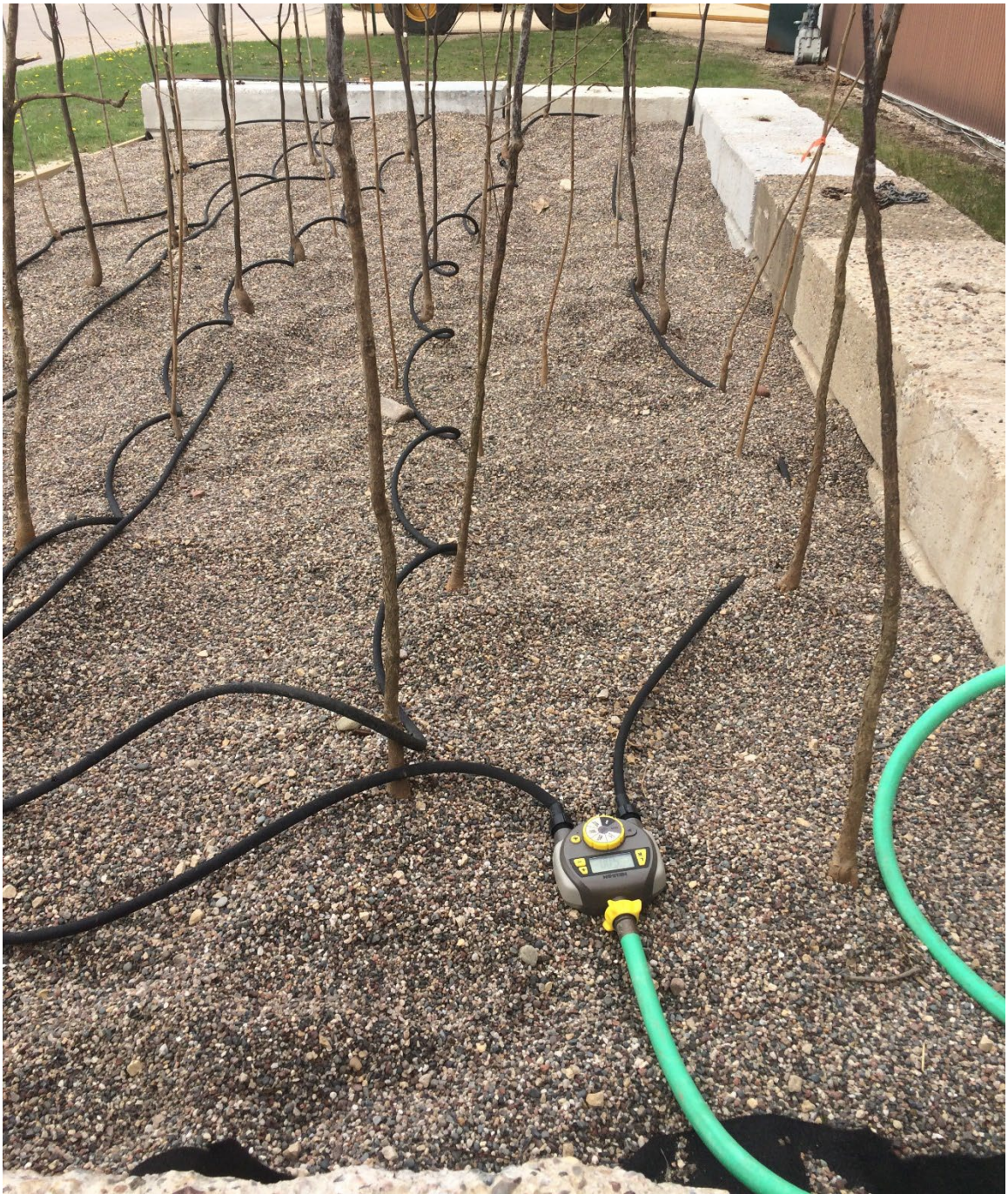
Soaker hoses are very popular with communities, inexpensive, and very frugal water users. This system is regulated by an inexpensive timer. Photo credit: J. Wahls.
