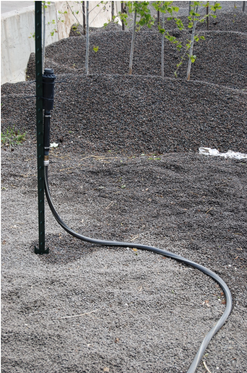
Inexpensive spray heads attached to fence posts in the bed with a garden hose supplying the water.
